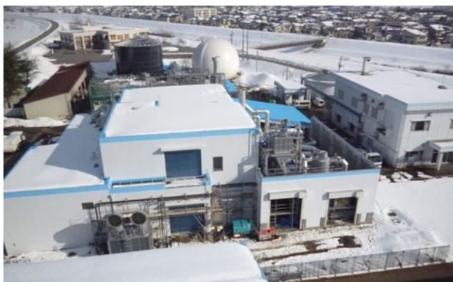
The facility to produce biogas from food scraps is under construction. (late January)
